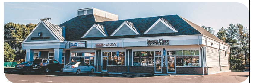
Mozzicato Retail, Rocky Hill, CT | 2014 | Renovation — 6,000 sq. ft.
